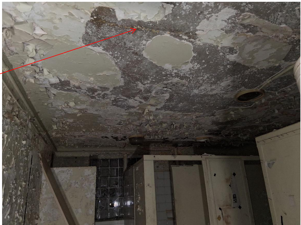
Fig. 4 – Fissure & Infiltration
