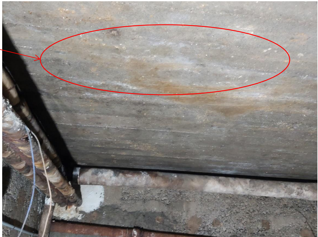
Fig. 3 – Infiltration
